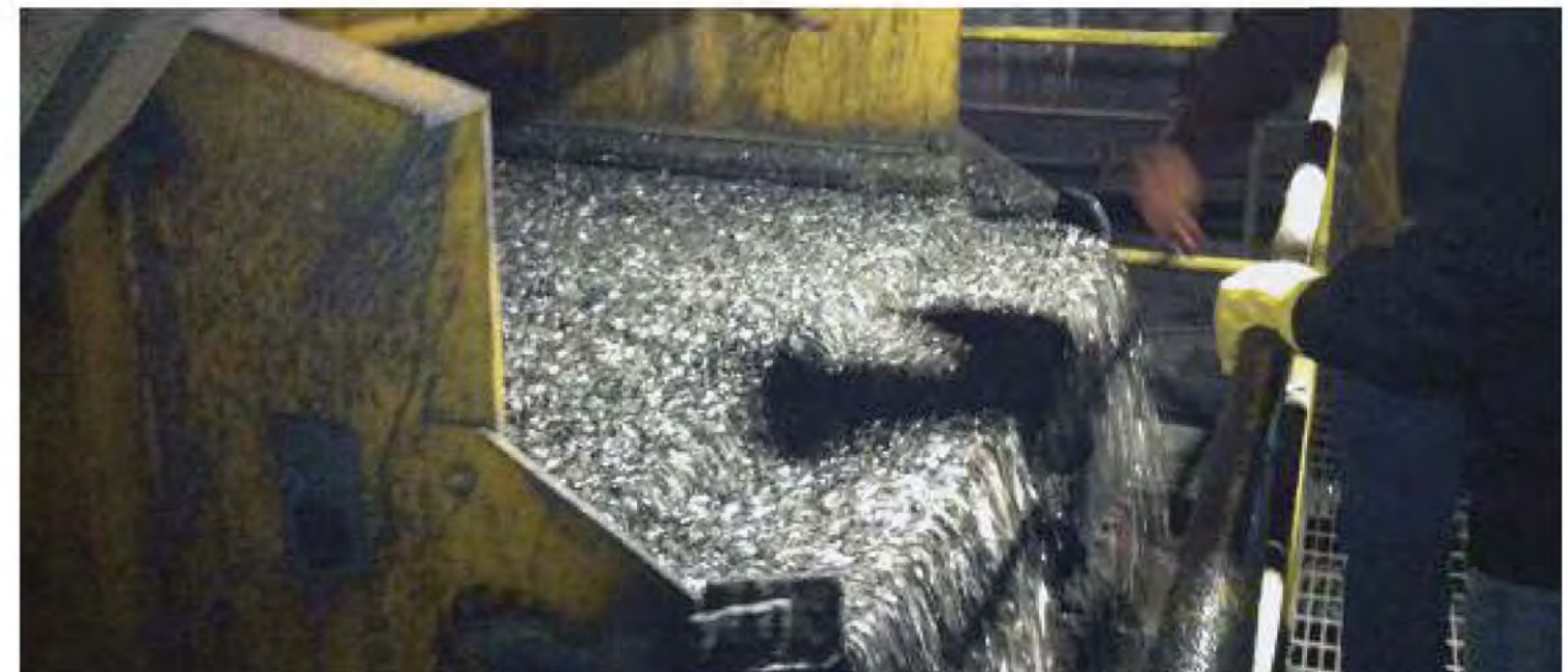
Coal flowing through the processing plant.
