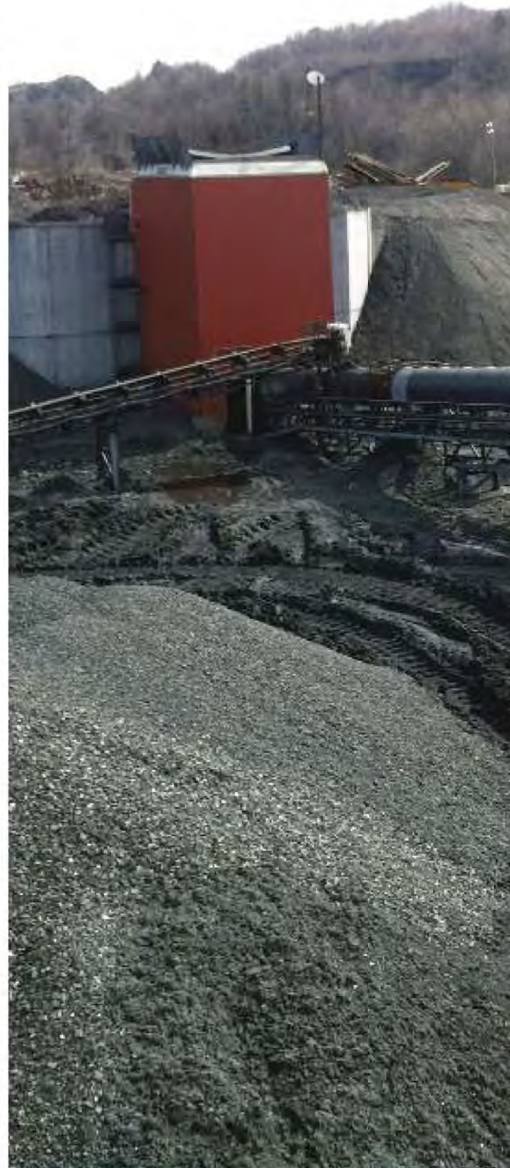
The red structure in the background is where the raw coal begins its journey through the New St. Nick breaker. Material is loaded at the top of the structure and the conveyor on the right feeds the breaker.
