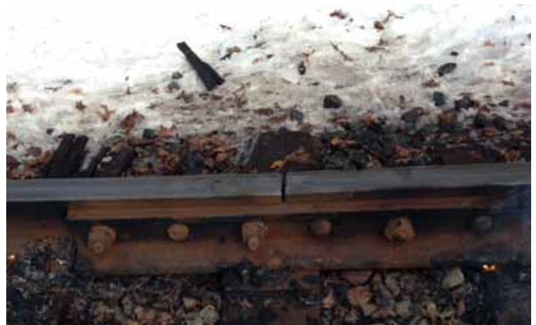
After being heated and repaired.
