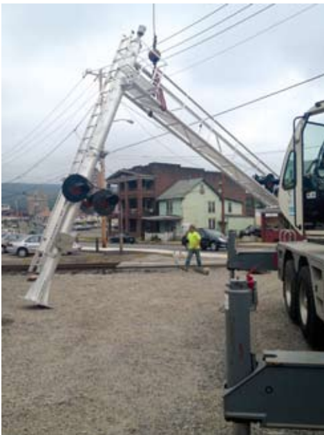
RBMN Signal Department installing new Cantilevers at the RT 309 road crossing in Tamaqua, PA
