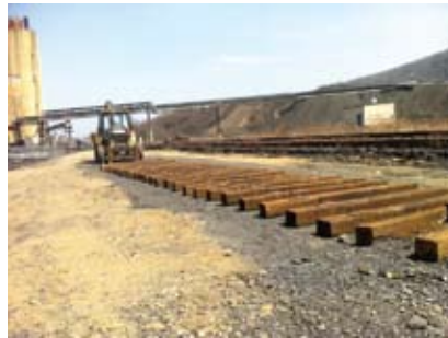
The Maintenance of Way Department has constructed a new rail siding for Reading Anthracite at the Gilberton coal facility
