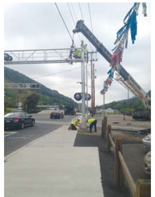
RBMN Signal Department installing new Cantilevers at the RT 309 road crossing in Tamaqua, PA
