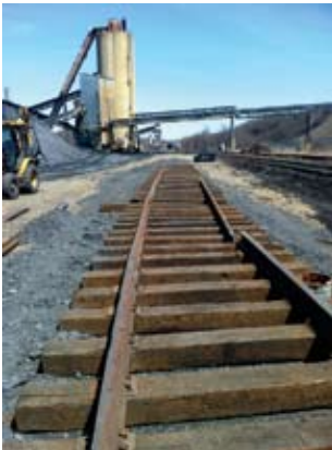
The Maintenance of Way Department has constructed a new rail siding for Reading Anthracite at the Gilberton coal facility
