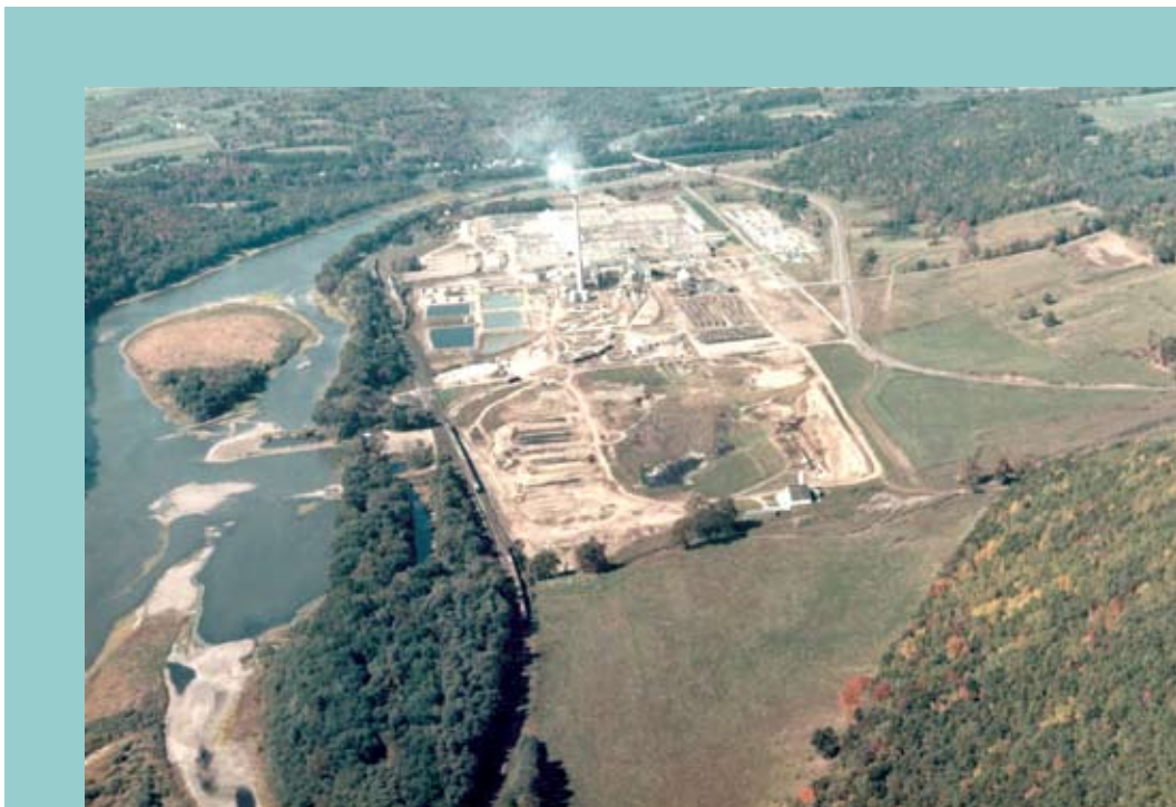
Aerial views of the Mehoopany plant, 1966(Left) and a current view (Right)
