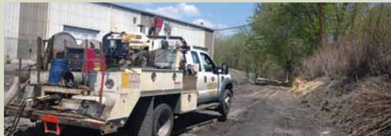
Dirt has been removed from the track and repairs started.
