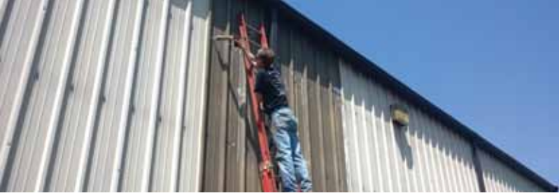
Filling holes in the warehouse wall.
