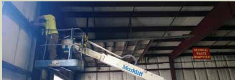
Electrical Systems being inspected and repaired.
