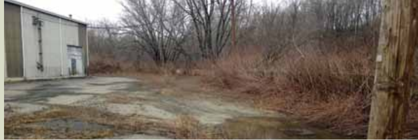
There is a track here – its buried under several feet of dirt.
