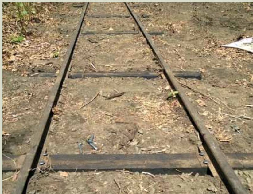
New ties installed.
