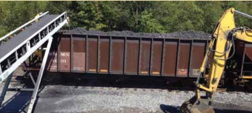
First loaded cars ready to be pulled.
