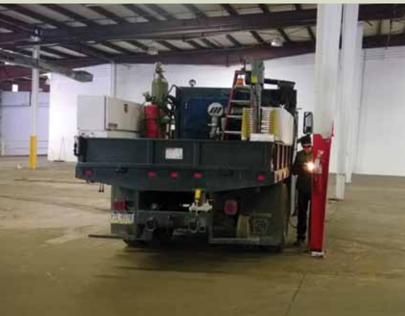
Jim Somers repairing interior support columns.
