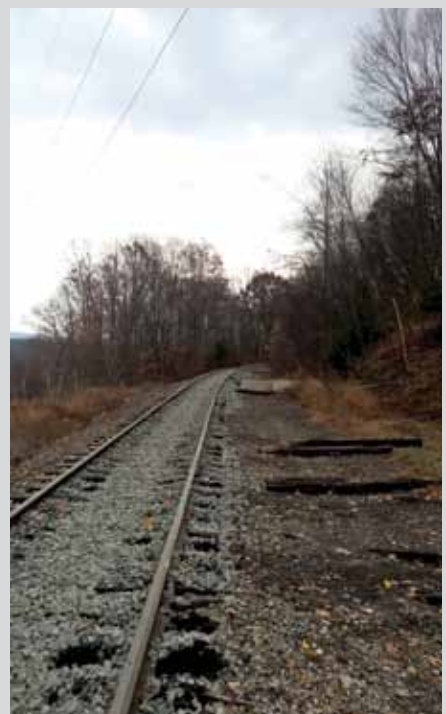
North end of curve on Hazleton line just north of Mauch Chunk Junction MP 0.63 before the ballast regulator completes the surfacing on a 3 inch raise.
