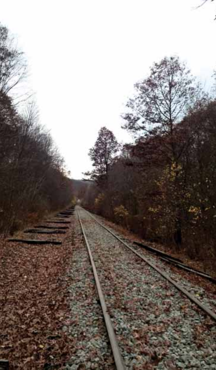
Freshly dumped ballast just south of Tamanend Road Crossing at MP 1.24 prior to being tamped and regulated for a finished look on the newly installed ties.
