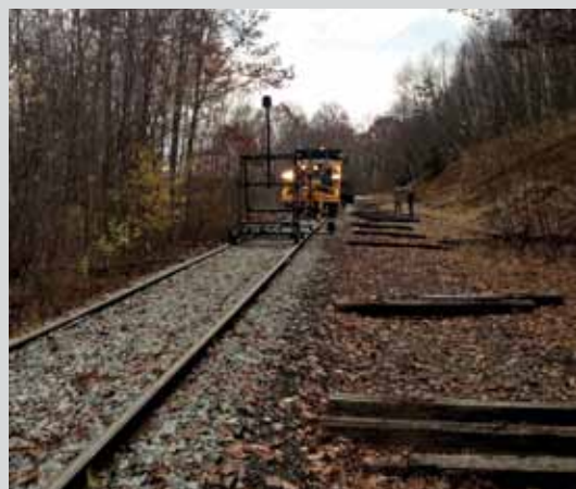
Mark IV with buggies out in front to raise 3 inches, line, and tamp the track. Tamper is following the tie work gang just north of Mauch Chunk Junction MP 0.63. Andy Muller and Justin Levan along the ROW watching John Brown work in the Mark IV.
