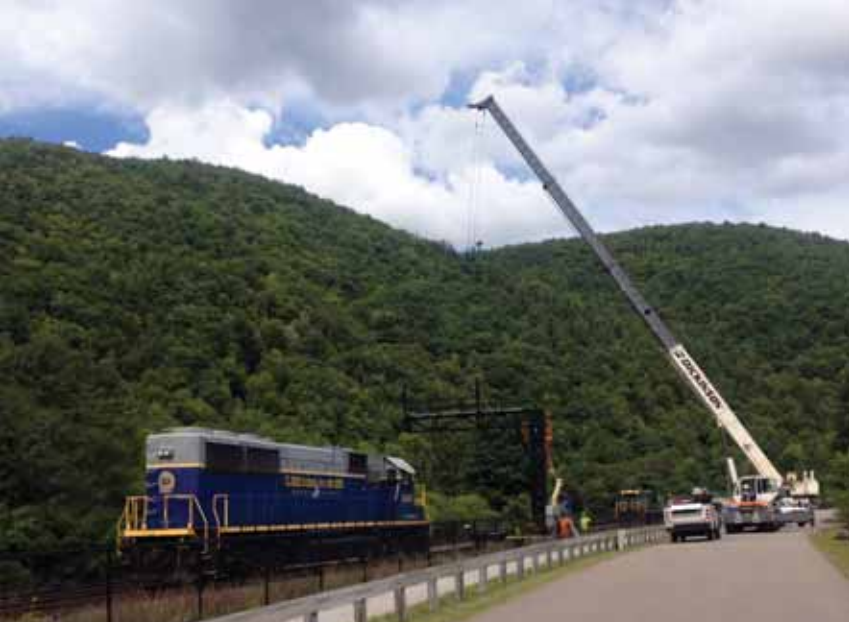
Cantilever re-erected at new site at Coal Interlocking.
