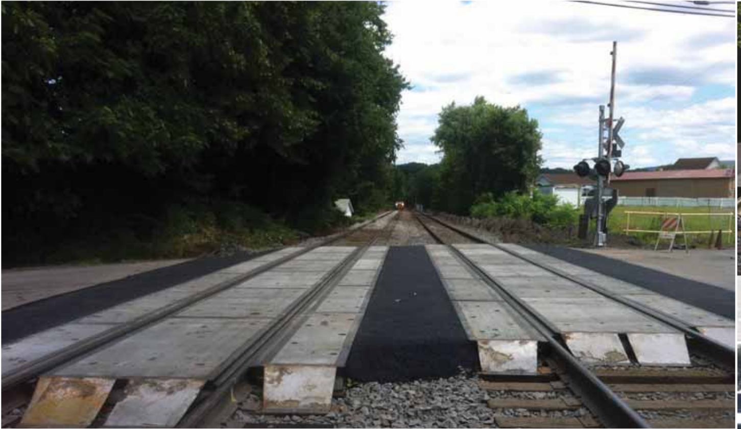
New concrete panels on tracks 1 & 2 at Main Street MP 175.19.
