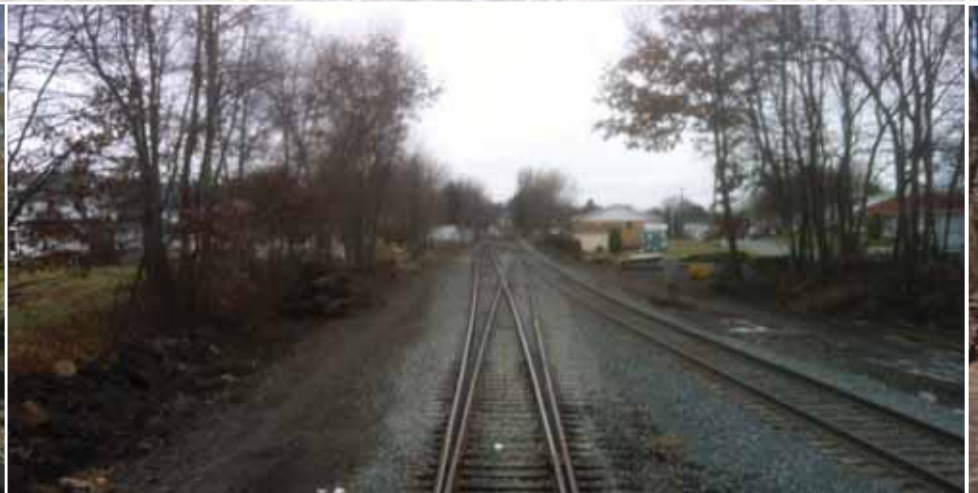
Standing on the Susquehanna branch looking south, marking out the layout of a new equilateral switch and realignment of tracks along with rehabilitating the crossover viewed in the far distance at Dupont MP 175.5
