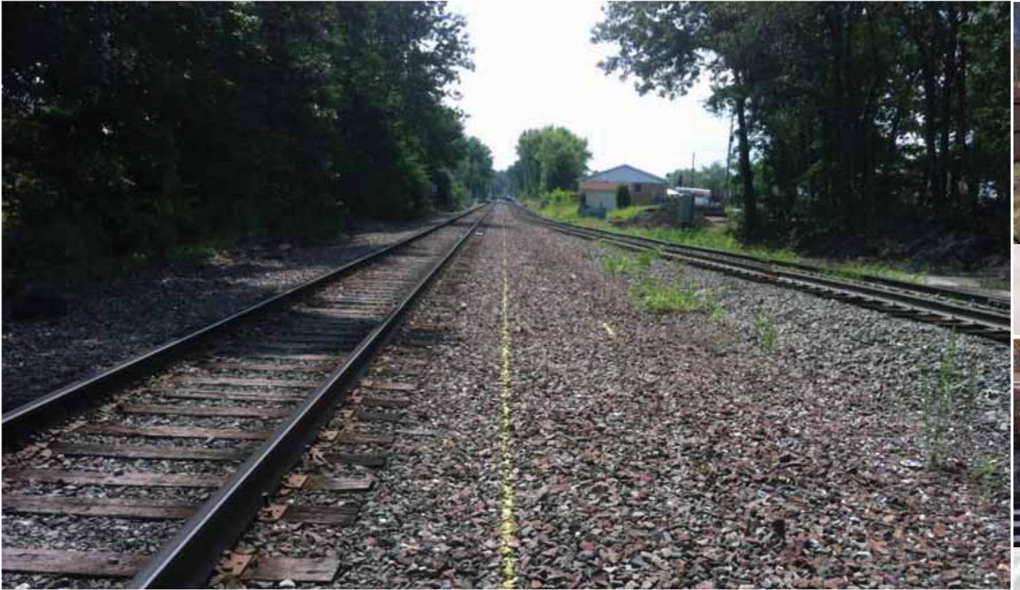
Standing on the Susquehanna branch looking south, marking out the layout of a new equilateral switch and realignment of tracks along with rehabilitating the crossover viewed in the far distance at Dupont MP 175.5
