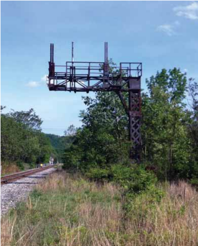
Cantilever at it's original location in Schuylkill Haven PA before any work or modification.
