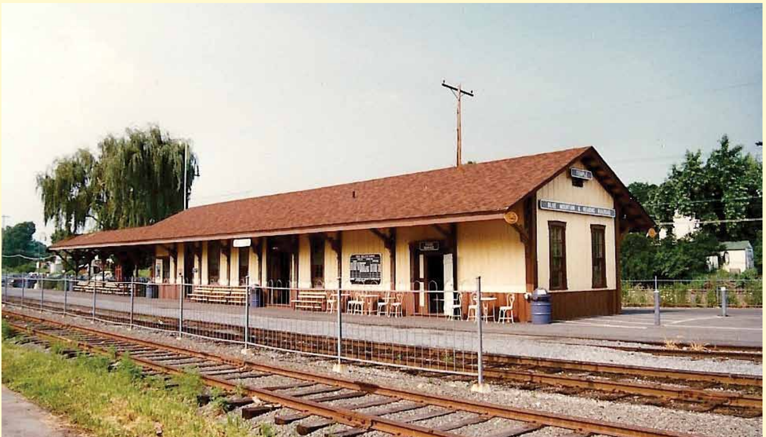
Temple Station after construction is finished.
