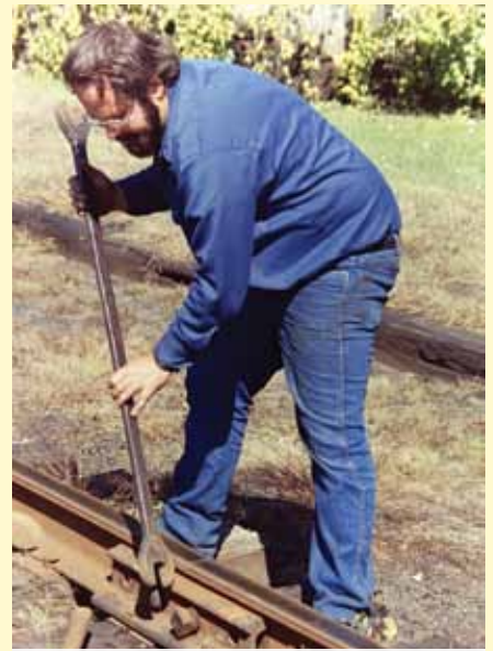
Mike Tilger tightening bolt on the Perkiomen Branch.
