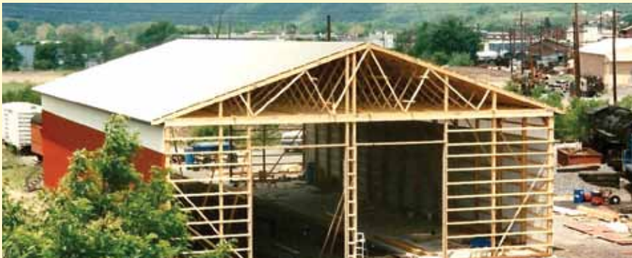
South Hamburg Engine House being constructed.
