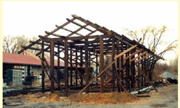
Temple Station while being constructed.
