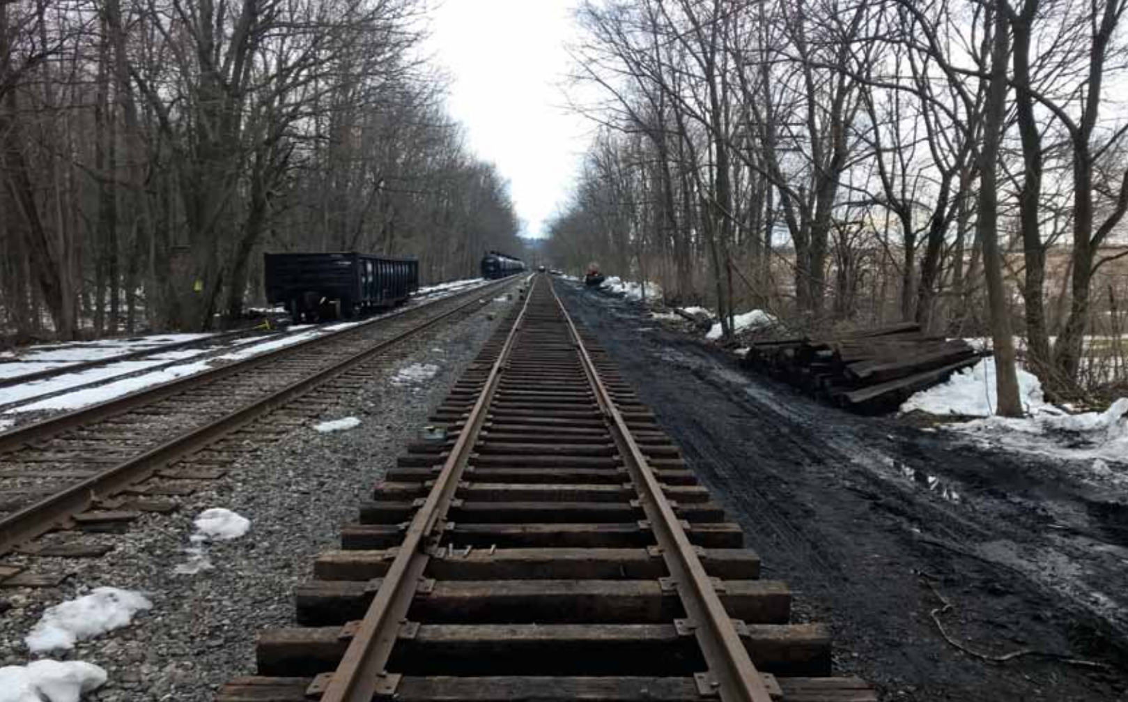
New track construction along the Mainline in Mohrsville, Pennsylvania.
