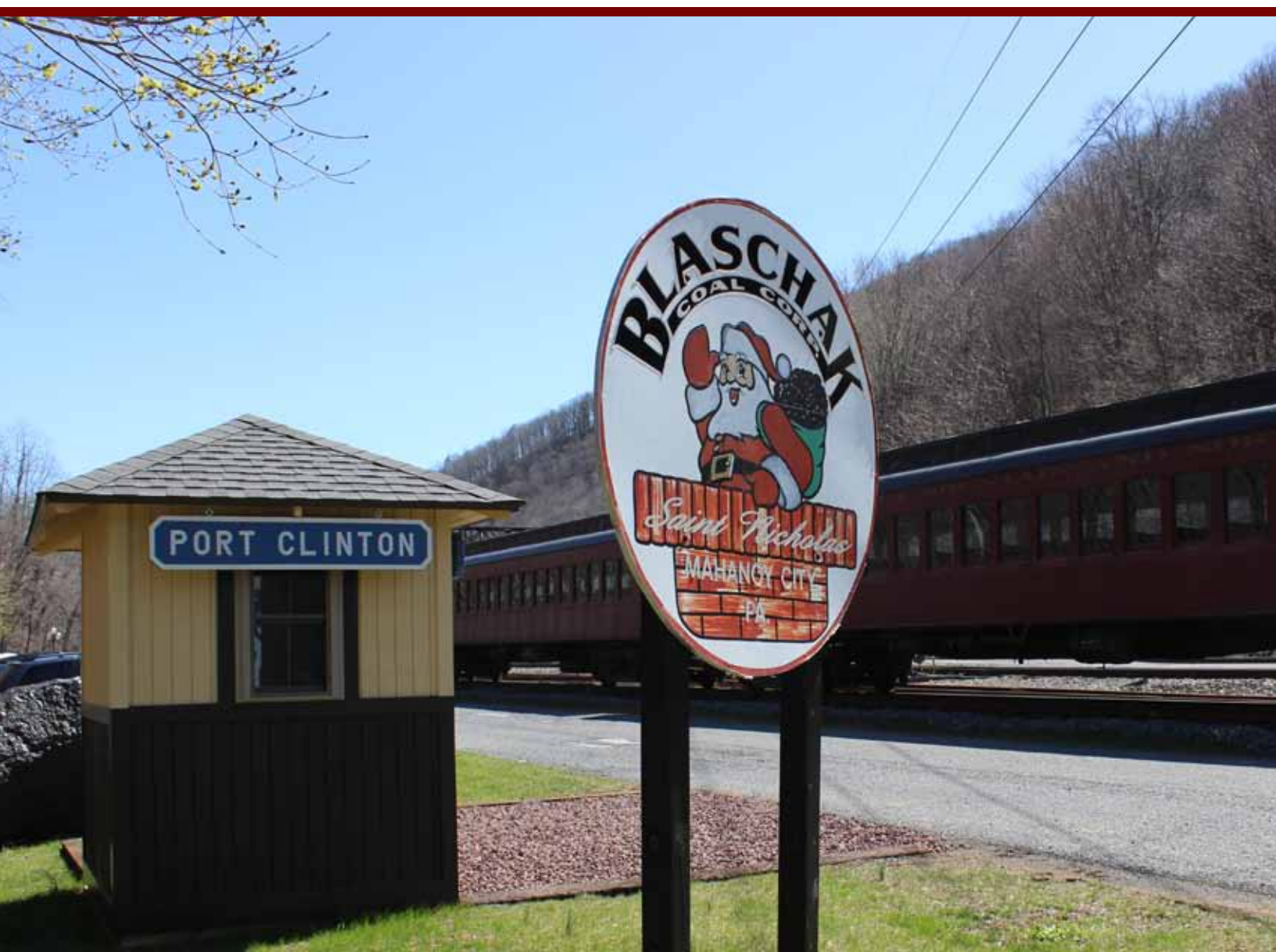
The newly constructed ticket booth at Reading & Northern Corporate Headquarters in Port Clinton.
