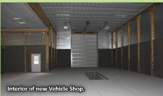
New Vehicle Shop at Port Clinton.
