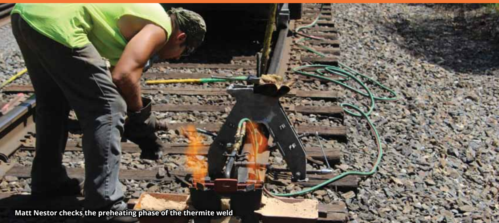
Thermite welders, Chris Orlick, Larry WellerIMG, and Matt Nestor are welding in the new rail string at MP 89.5
