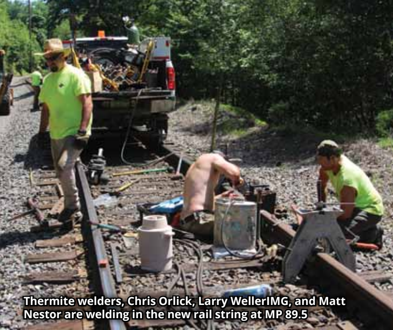
Matt Nestor and Larry Weller carry the welding shears into position as Chris Orlick starts the torch to drop a weld on new rail MP 89.5
