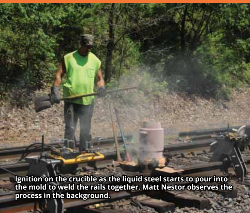
Matt Nestor checks the preheating phase of the thermite weld
