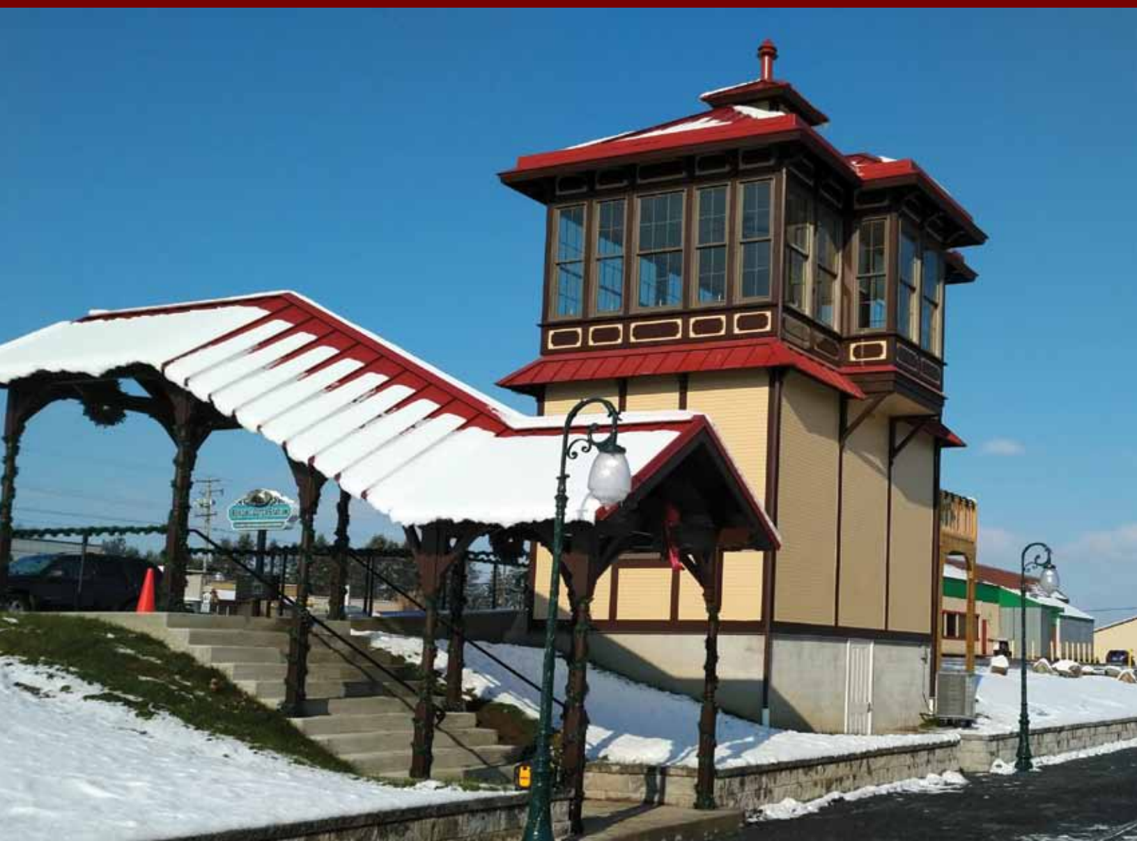
View of the Outer Station tower from the newly laid platform looking north on the Reading & Northern Main Line. For excursions out of Outer Station visit our website www.rbmnr-passenger.com .
