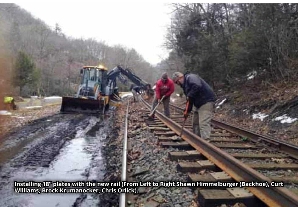
Replacing rail on our Minersville Track (Larry Weller, Curt Williams, Chris Orlick).
