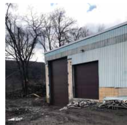
New garage doors at Ransome Warehouse
