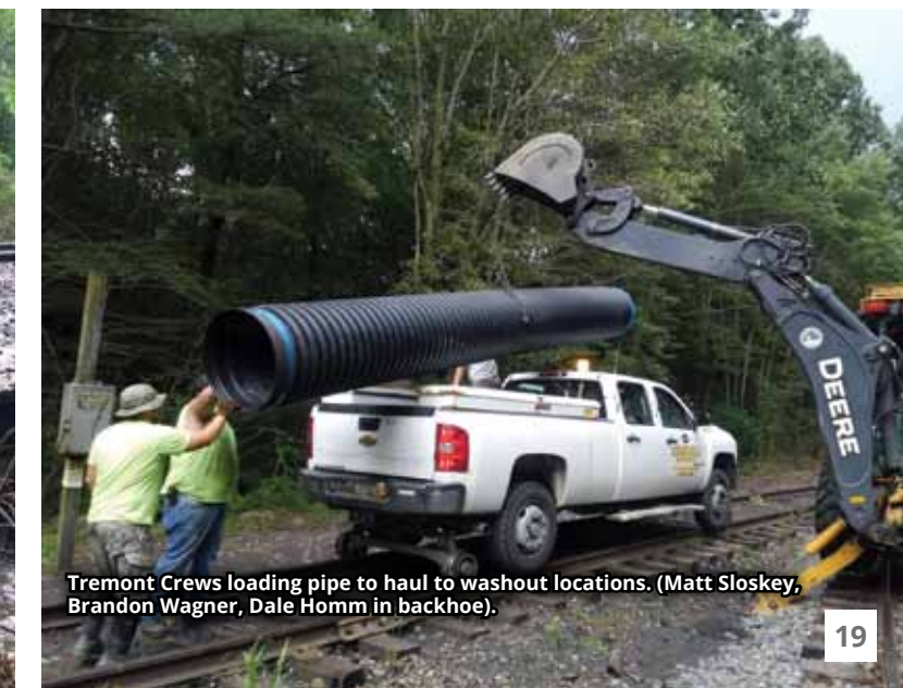
Tremont Branch washout repaired with new pipes installed along with large rocks to prevent the erosion of our banks.
