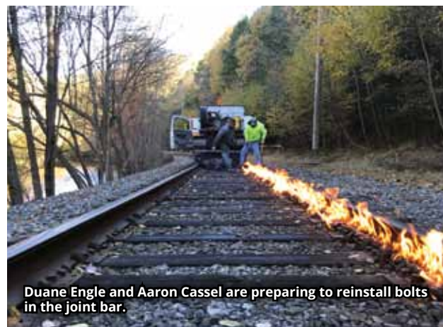
Duane Engle utilizing FIRESNAKE to heat the rails so the rail can "grow" back together.
