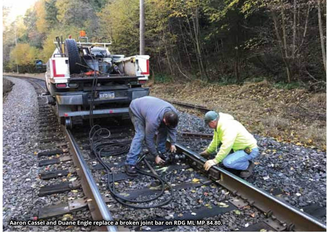
Aron Cassel and Duane Engle replacing broken joint bar. During this process, the rails pulled apart due to cold temperatures.
