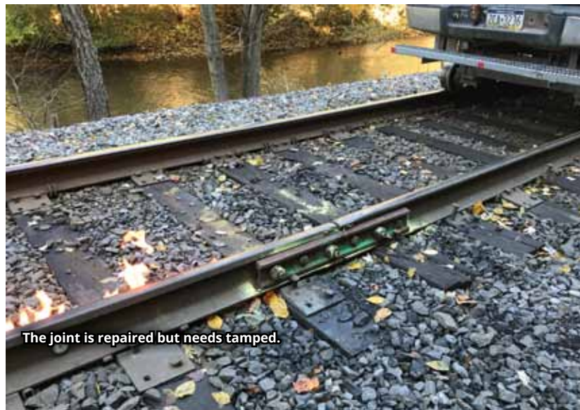
Aron Cassel closely monitoring the FIRESNAKE to ensure the rail is expanding.
