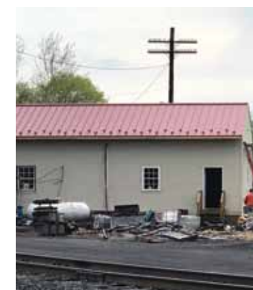
Pittston Yard Office Addition
