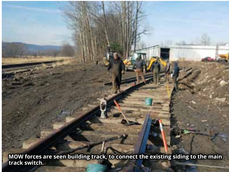
Matt Minnich, Shawn Slusser, and Josh Rodney are spiking track, as Duane Zimmerman passes in the background.
