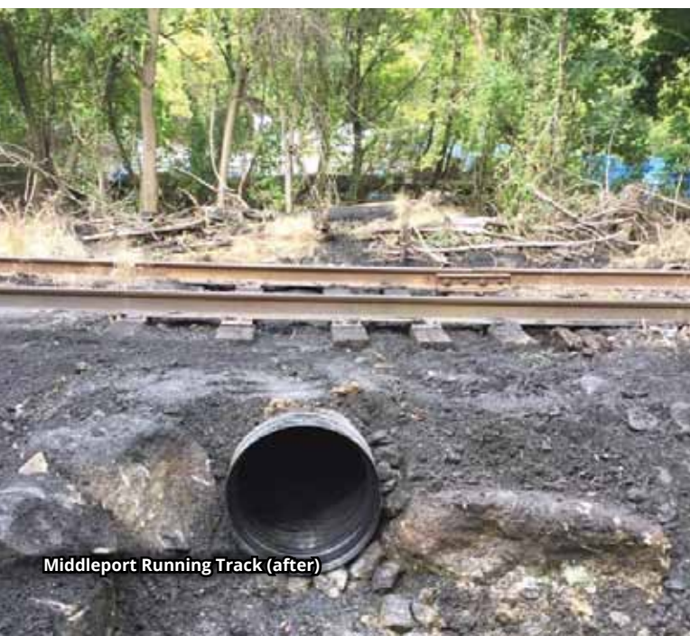
Tremont Branch installing additional pipes adjacent to our culverts to prevent another washout.
