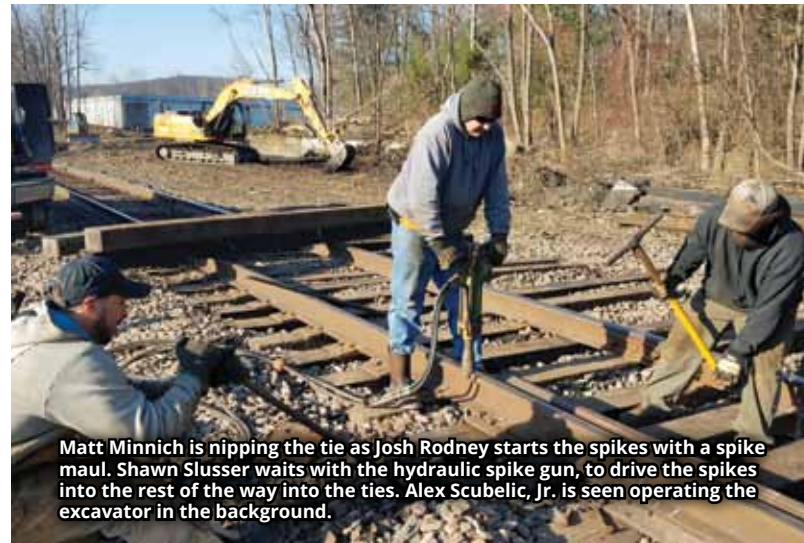
MOW forces installed this new switch at Ransom to reconnect the warehouse siding to the main track. The switch was installed in only five days.
