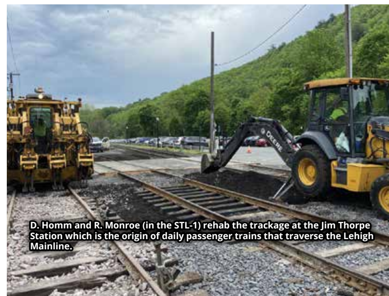
A photo of a TKO recently this year installing new ties at Lehigh ML MP 124 by R. Monroe.
