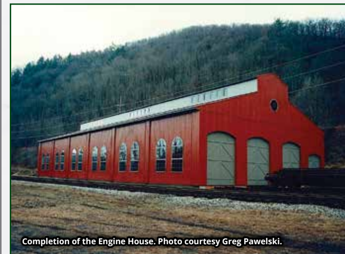
Frame of the now existing Engine House - with a building-free background in Port Clinton. Photo courtesy Greg Pawelski.
