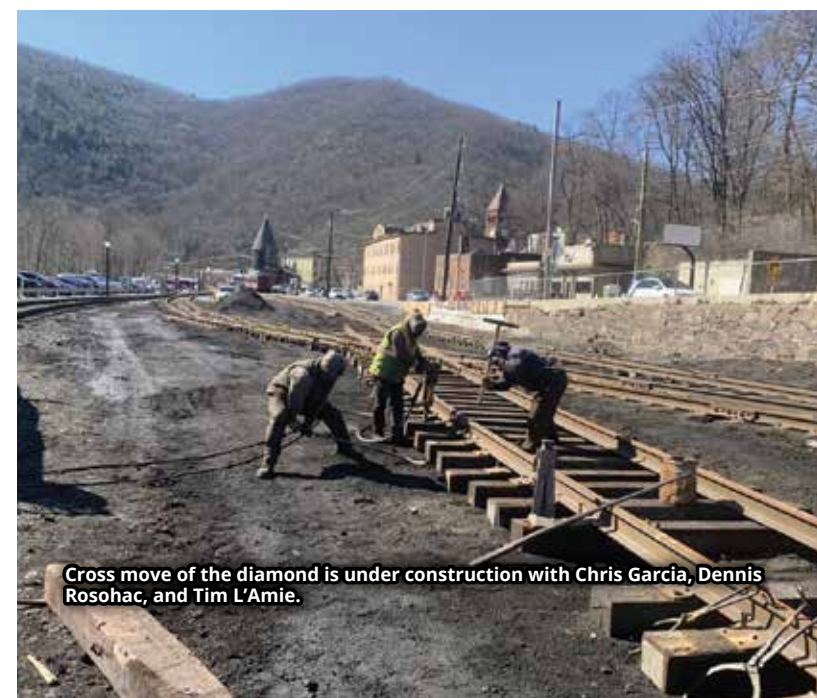
Included with the Jim Thorpe rehab was the install of a diamond being facilitated by Dennis Rosohac, Dave Hutton, and Chris Garcia.
