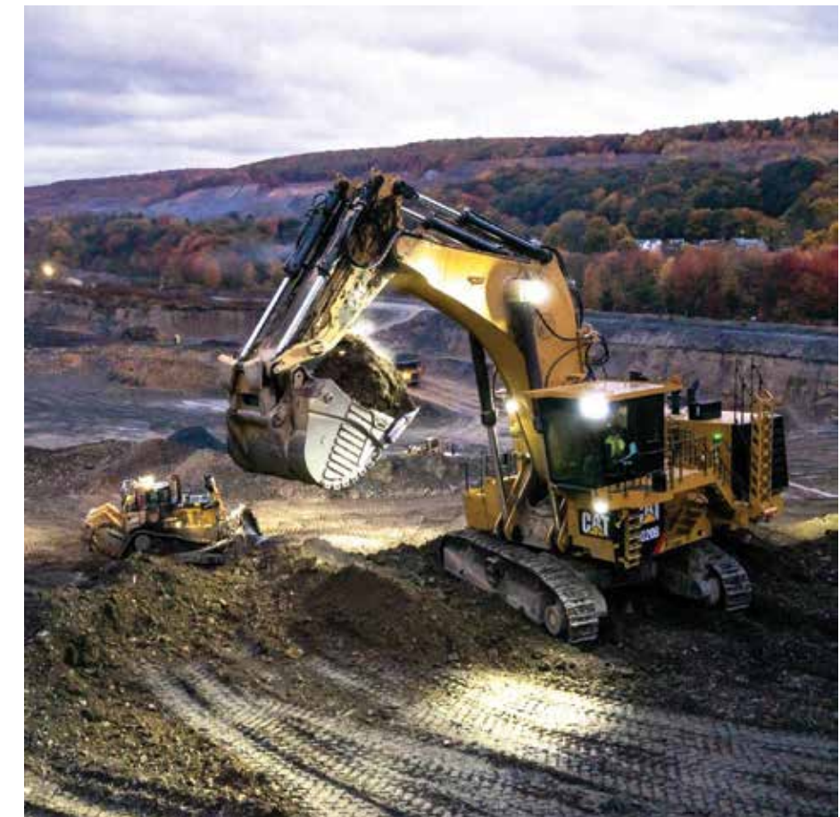
A Caterpillar excavator and large bulldozer work in tandem at one of Reading Anthracite's various strip-mining sites to remove overburden as they work towards the coal seam.
