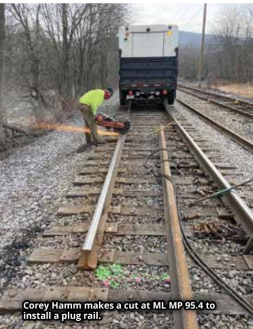
Corey Hamm makes a cut at ML MP 95.4 to install a plug rail.
