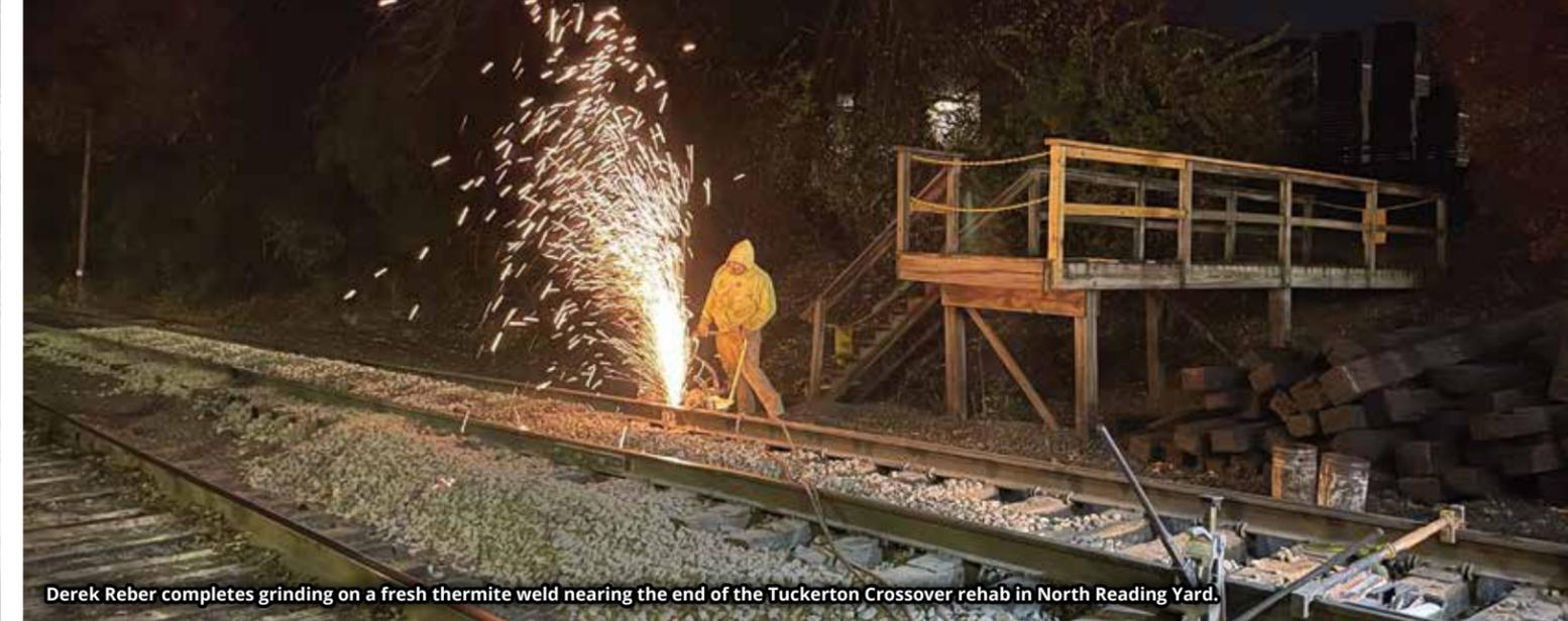
Derek Reber completes grinding on a fresh thermite weld nearing the end of the Tuckerton Crossover rehab in North Reading Yard.
