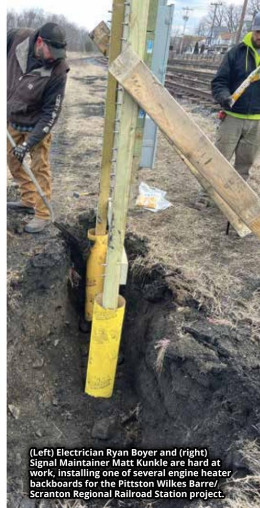
(Left) Electrician Ryan Boyer and (right) Signal Maintainer Matt Kunkle are hard at work, installing one of several engine heater backboards for the Pittston Wilkes Barre/Scranton Regional Railroad Station project.
