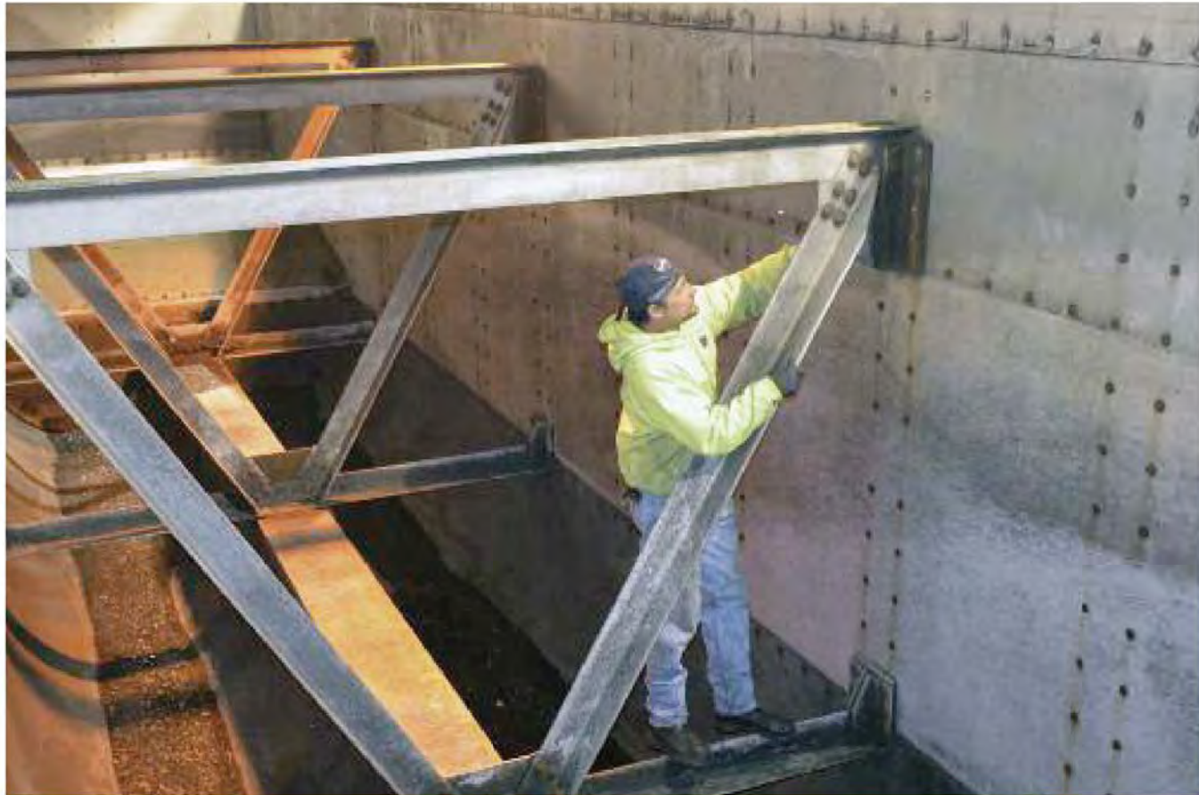
Jim Somers replacing a bolt inside of an aluminum coal car.
