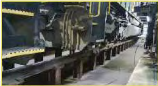
The Inspection Pit.
