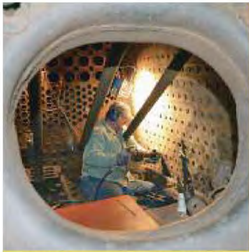
Shane Frederickson tightening the bolts from inside the firebox of the 425.
