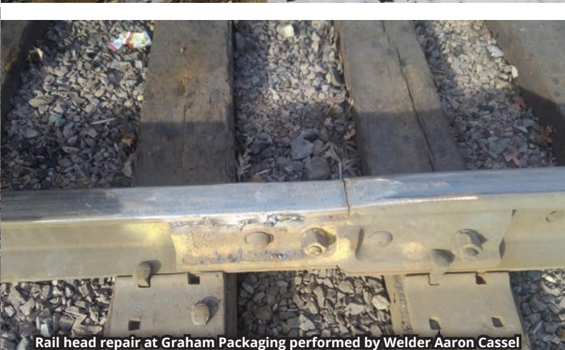
Rail head repair at Graham Packaging performed by Welder Aaron Cassel (After).
